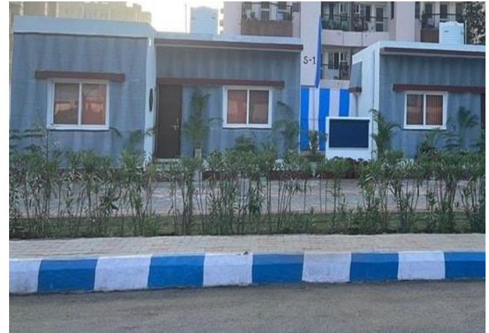
3D printed house built by Indian Army's MES in Gandhinagar.
